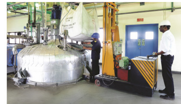
Raw material charging in progress.
